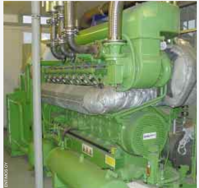
The engine consumes the wood gas, hence producing 2 MW of electric power.
